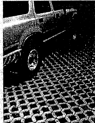
One type of alternative paver consists of a concrete lattice structure for support with grass growing in the void spaces. (Source: Lo Gioco Landscaping, Inc., no date)
